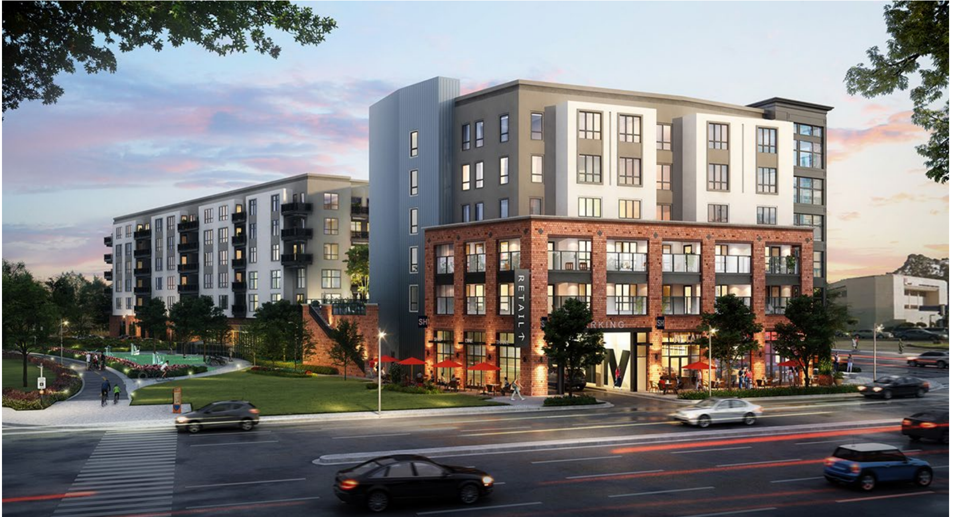
Source: KTG Architecture + Planning (SummerHill Apartment Communities, San Francisco)
