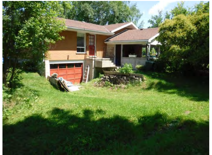
Plate 10: Garage attached to the basement with driveway ramp, facing north (Photo 7872).
