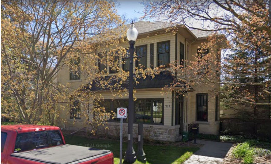
Figure 20: 210 St. Andrew Street E at present (Google, 2022)
