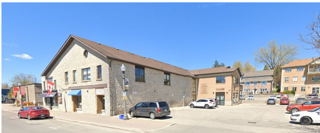
Figure 18: 181 St. Andrew Street E at present (Google, 2022)
