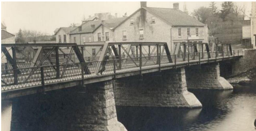
Historic Victoria Street Vehicle Bridge
