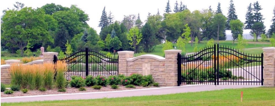
Figure 27: Christ the King Cemetery Entry Feature and Planting Bed. Design/ Photo: HLI
