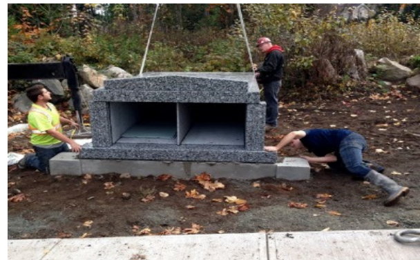
Installation of double lawn crypt
