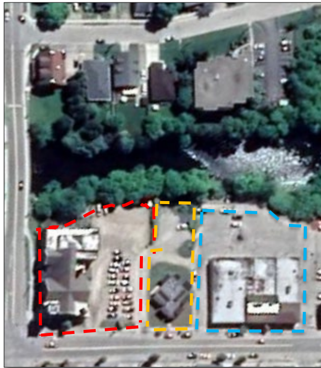
Figure 29: Aerial of 300 (in red), 350 (in yellow) and 380-398 (in blue) St. Andrew St W (Source: Google maps)
