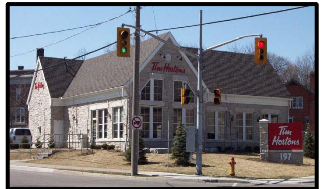
Figure 6.5: The peaked roof of this low-rise building screens all rooftop equipment and helps define the intersection where the building is situated.
