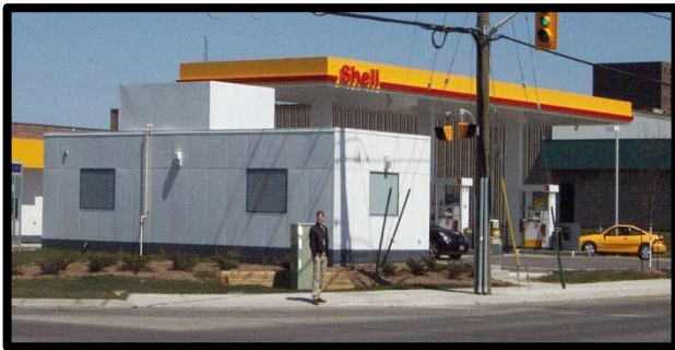
Figure 6.7: Although the rooftop equipment on this gas station is fully screened with materials matching the building, the enclosure is not well-integrated with the building form.
