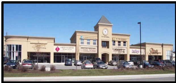
Figure 6.3: Rooftop equipment screening methods used on this building include parapets, an articulated roofline, and centralized location of equipment.
