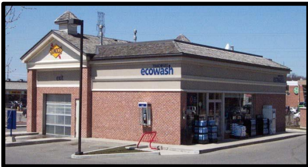
Figure 6.8: The articulated roofline on this gas station and car wash fully screens rooftop mechanical equipment and helps create an attractive building design.
