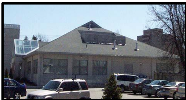
Figure 6.4: Rooftop mechanical equipment for this building is hidden by a screening wall that is integrated
