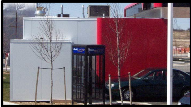
Figure 6.6: The rooftop equipment on this corner gas station is not screened and is visible from public view.
