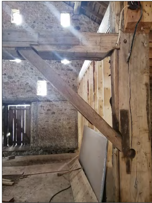
Figures 25 & 26- (above) Detailed view of stone slit opening construction from interior; (below) View of mortise and tenon construction in the interior of the barn (Source: MHBC, 2022).
