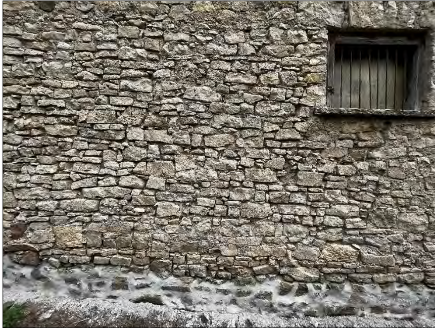
Figure 37- Detailed view of rubble stone facade (Source: MHBC 2022).
